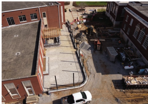
The outdoor dining area will be complete this spring.
