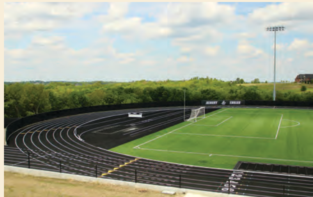
The Outdoor Venue project is now in Phase II of construction.
